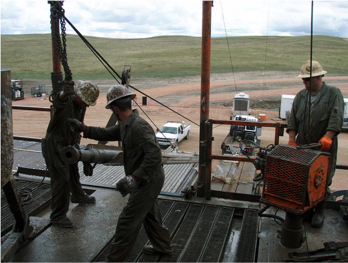
Figure 2-6. Pulling drill pipe onto the drilling platform.
