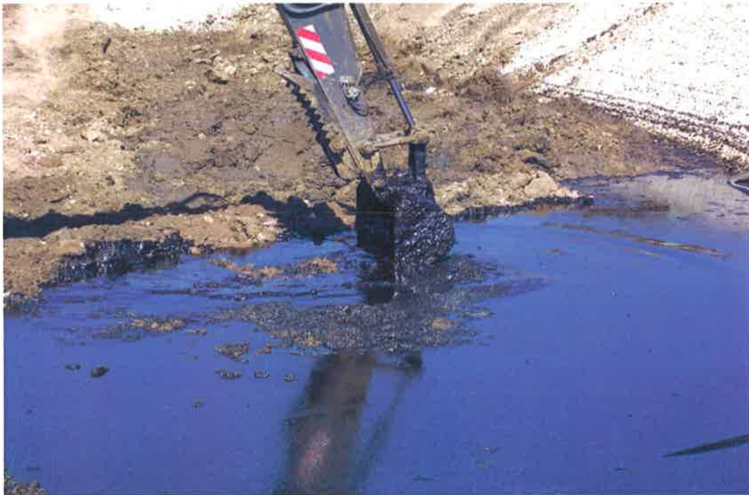
PHOTO 5 - RECOVERY OF RELEASED PRODUCT WITHIN TANK 303 CONTAINMENT
