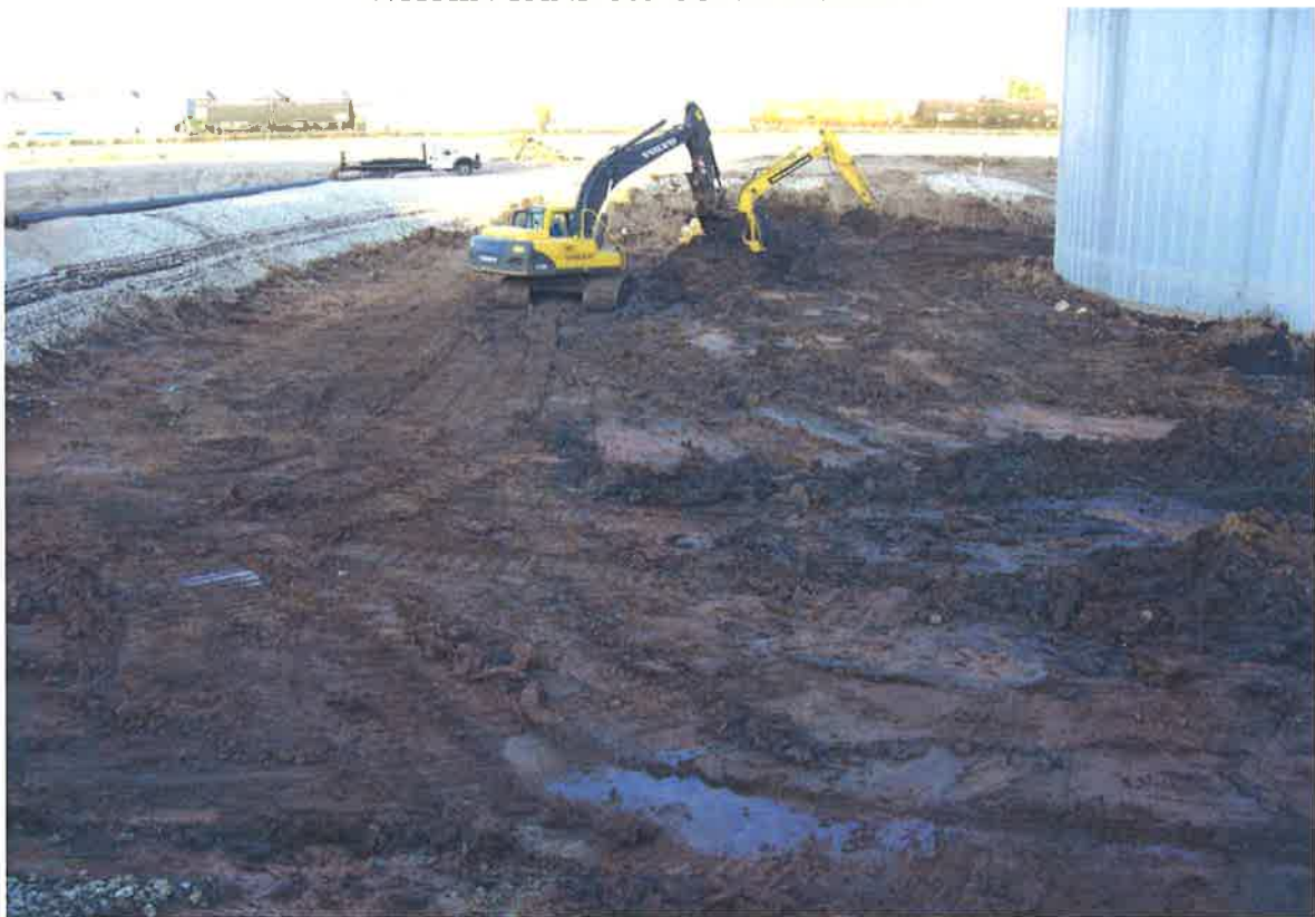
PHOTO 8 - SCRAPING OF TANK 303 CONTAINMENT BOTTOM
