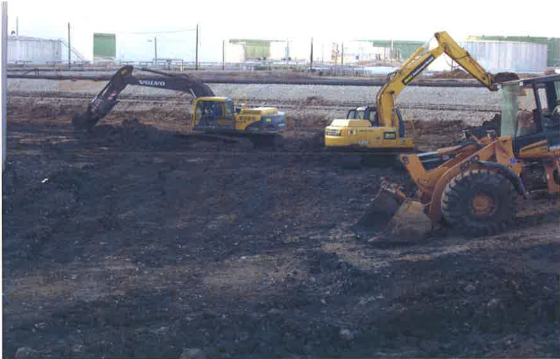
PHOTO 7 - SCRAPING AND MIXING OF IMPACTED SOILS WITHIN TANK 303 CONTAINMENT
