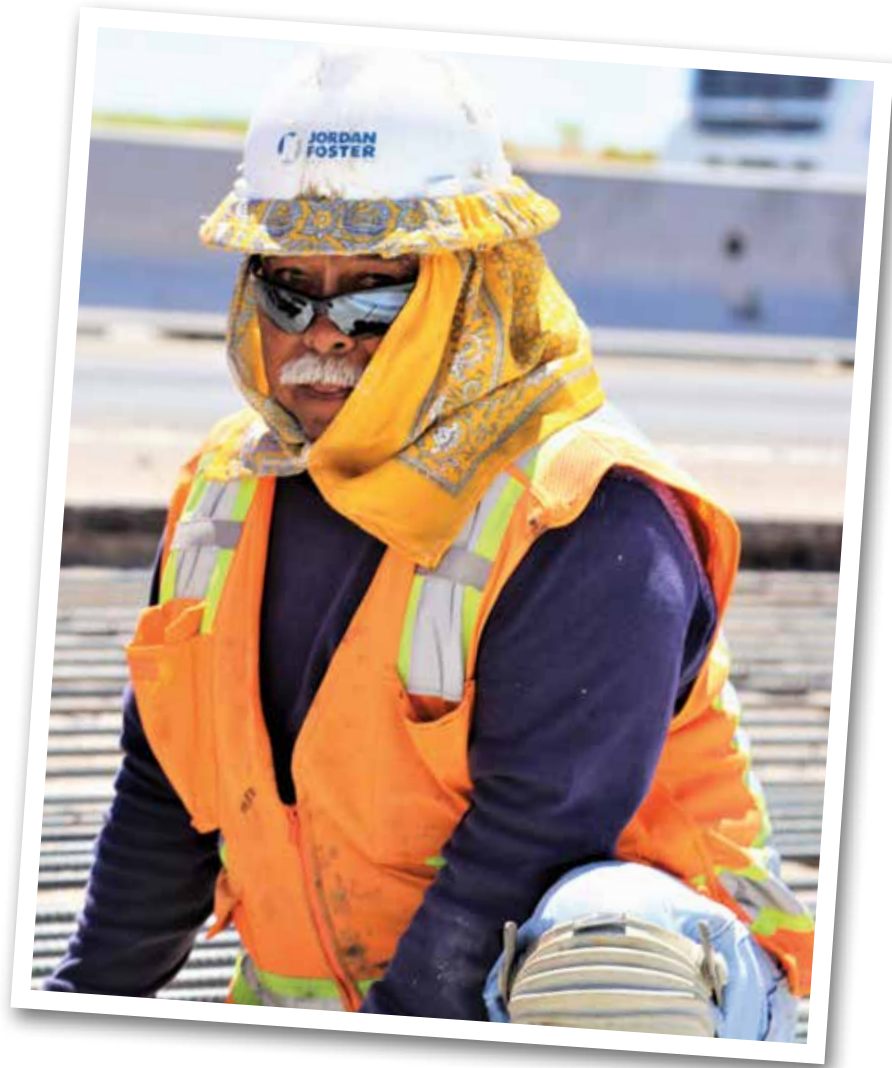
El Paso concrete finisher Leonardo Rodriguez (Jordan Foster Construction) dresses for the blazing sun.
